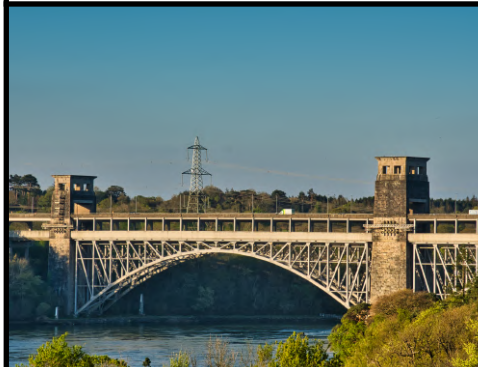
Britannia Bridge, Wales
